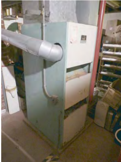
Example of older oil-fired warm-air furnace
