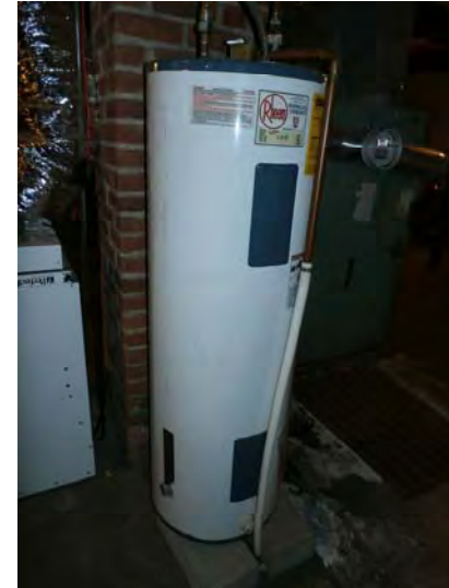
Typical electric water heater
