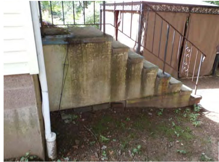
Typical larger pre-cast concrete stair stoop
